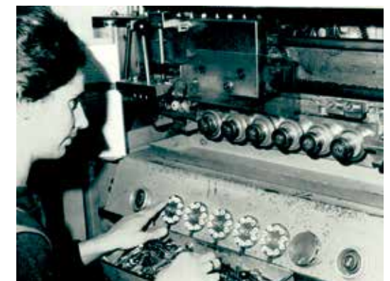
Setting up of a key cutting machine
